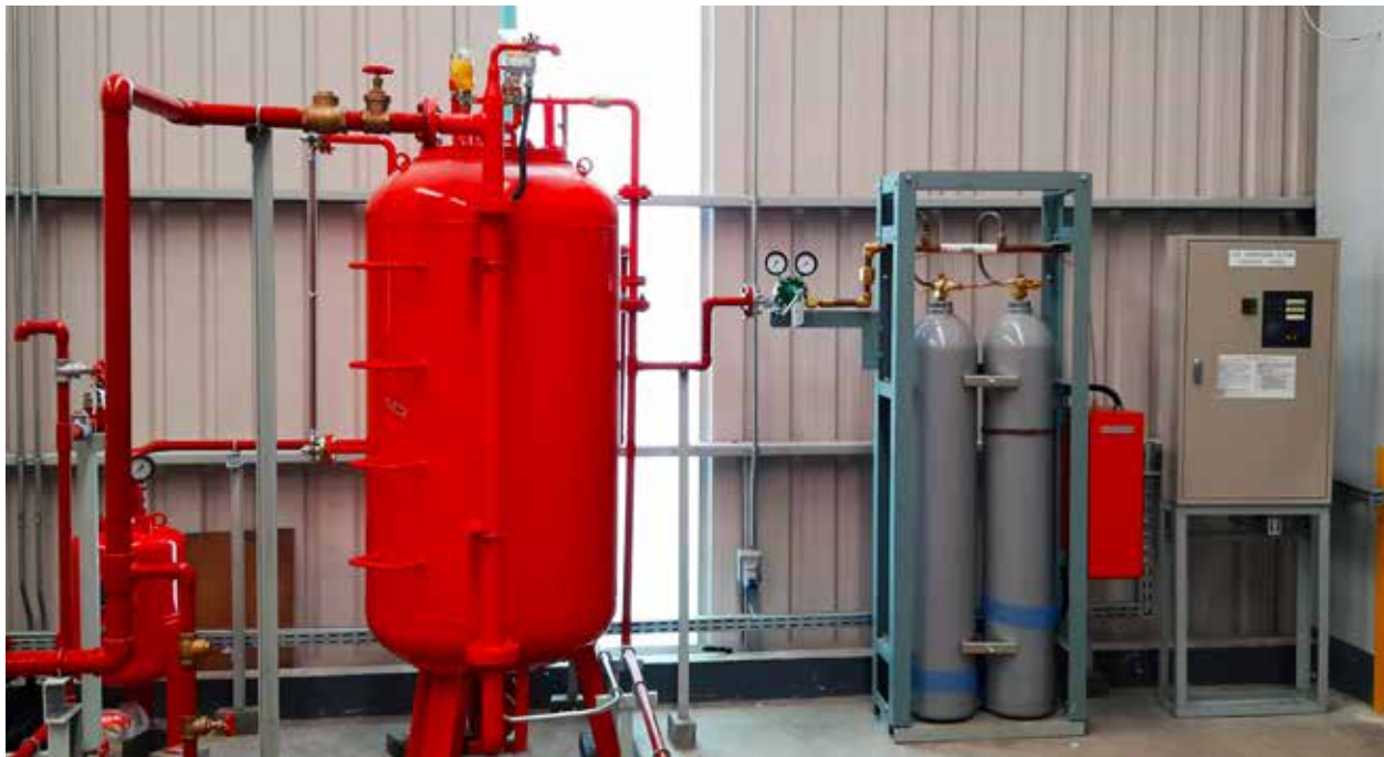
Nohmi Foam Extinguishing System, High Expansion ■
